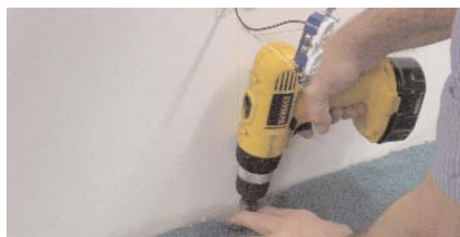
DRILL 1/2" HOLE PARALLEL TO WALL THROUGH FLOOR WHERE VERTICAL LINE FROM OUTLET MEETS FLOOR.
