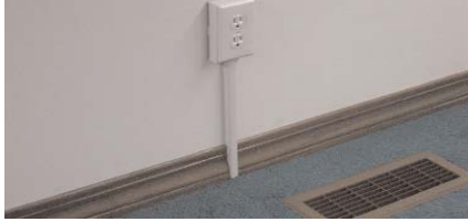
FINAL SURFACE WIRING INSTALLATION WITH ASLL.
