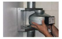
2. Mount Easy Flip™ chassis in an accessible location and connect duct to 4" collars.
